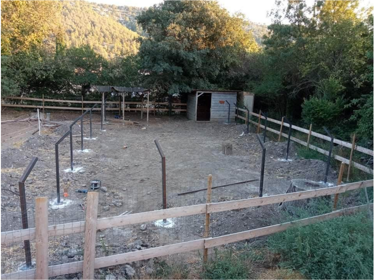
Figure 8: Enclos en construction
